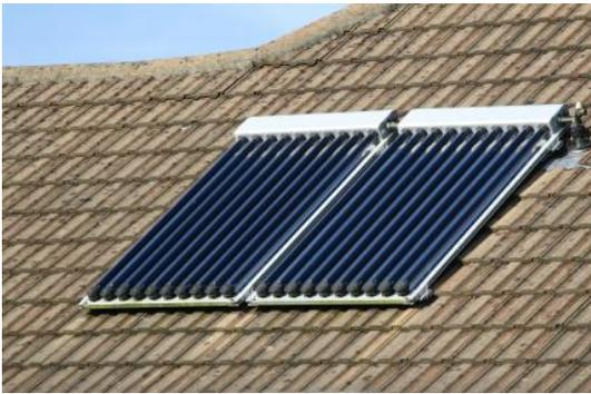
Figure 7 – Example of Solar water heating system with solar collectors<sup>8</sup>
